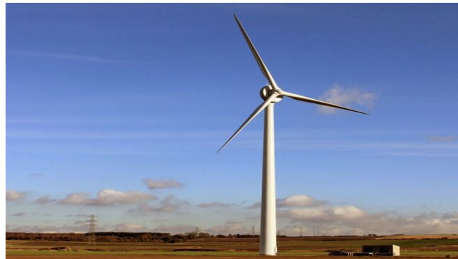
EWT DW52 900kW Turbine - Hub height: 40-50 m
