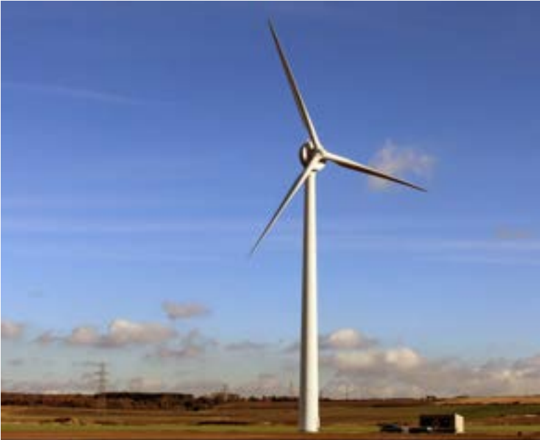
EWT DW52 900kW Turbine - Hub height: 40-50 m
