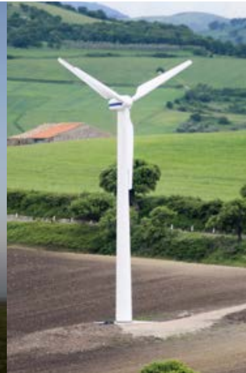
Endurance X-29 225kW Wind Turbine
